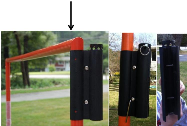
Use self-tapping screws and a Phillips head screw driver or electric drill to attach clamp to the goal uprights. It is easier to set the screws. It is easier to screw into if goal is laid face down. Be careful not to put all the weight on the clamps. This may cause them to shift out of the desired angle.
